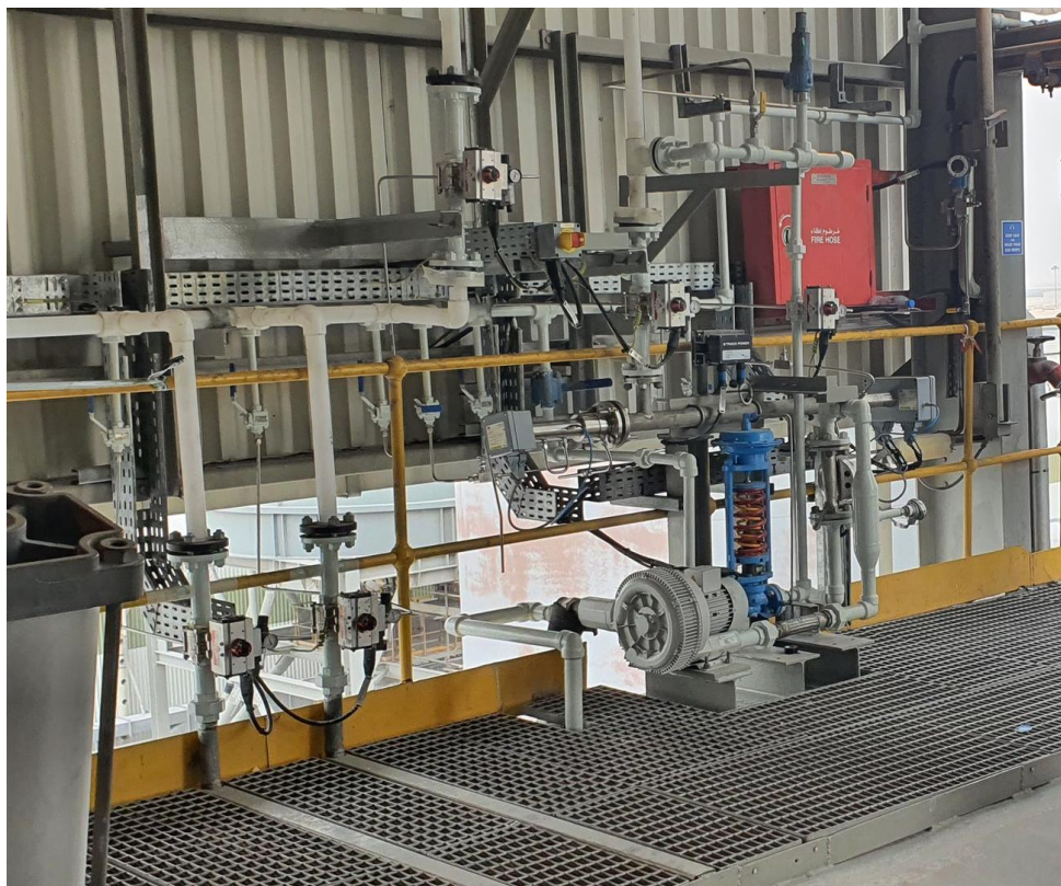
Figure 5. Sniffer system installation at GTC filter top level (inside penthouse).
